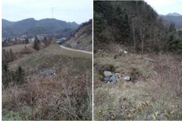
弃渣场绿化和挡土墙
