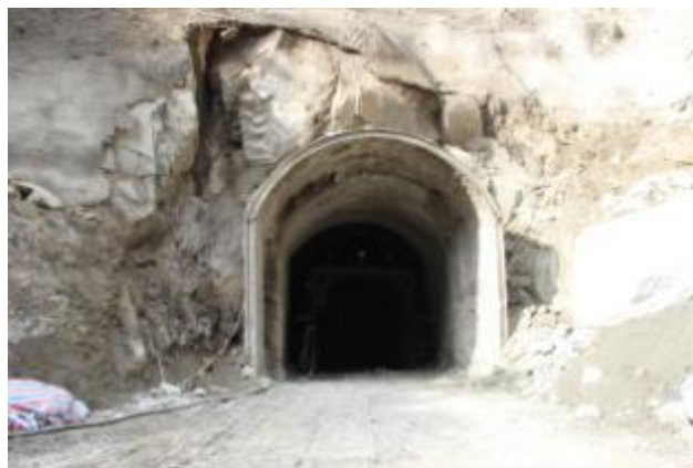
1#支洞洞脸支护及高边坡喷锚支护
